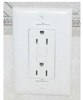
Figure 7-5. Typical AC Receptacle
