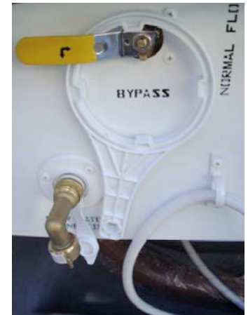
Figure 11-8. Water Heater Bypass System
