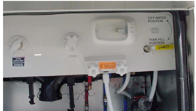
Figure 11-6. City Water Connection
