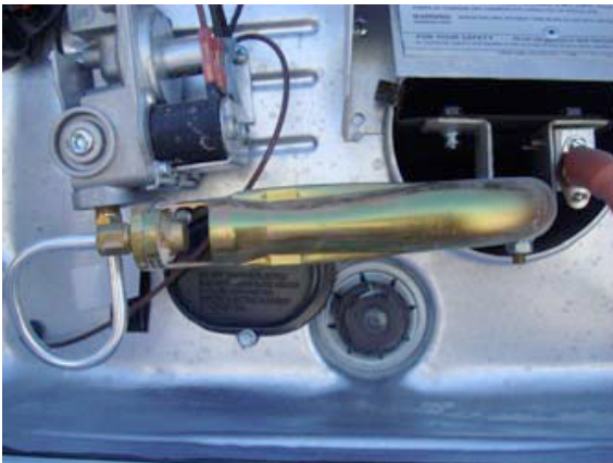
Figure 4-13. Water Heater Drain
